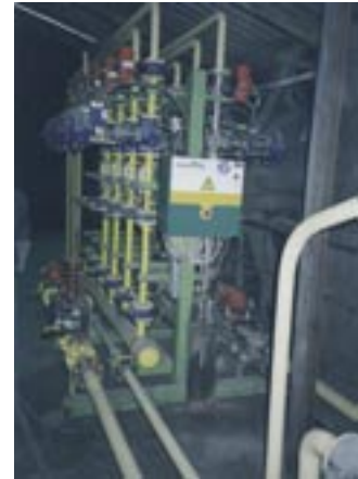
The oxygen/gas valve train is safe, compact and reliable.
